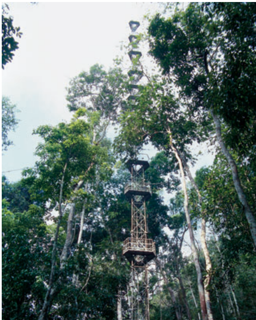
Observation tower for meteorological and carbon flux measurements near Xishuangbanna Station(23), ZHAO Shidong
